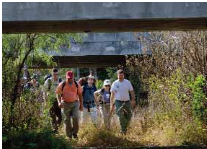
Accompanied on foot by a group of public land and resource managers and state wildlife biologists, the expedition passes beneath I-75 through one of thirty-six wildlife underpasses specially constructed when the former two-lane "Alligator Alley," which bisects the Florida Everglades, was converted to an interstate highway. PHOTO: © CARLTON WARD, JR.
