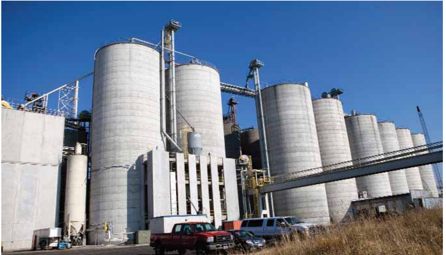
A row of grain silos at the Didion Milling company's ethanol plant in Cambria, Wisconsin, which also makes dried distiller grains as a byproduct that are used for animal feed.
